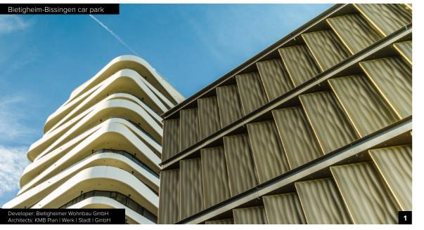
1 The envelope of the Bietigheim-Bissingen car park was manufactured using modern production processes. The facade panels are edged on all four sides. The solid undulating aluminium sheets are anodised in a bronze tone and mounted vertically as standing slats in the facade. Solid aluminium sheet | Elox, C32 | Wave
